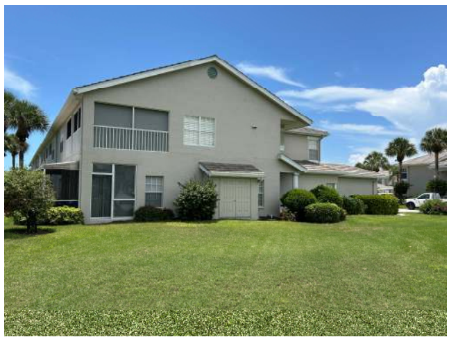
ROOF GEOMETRY – Gable / Other Roof Shape
