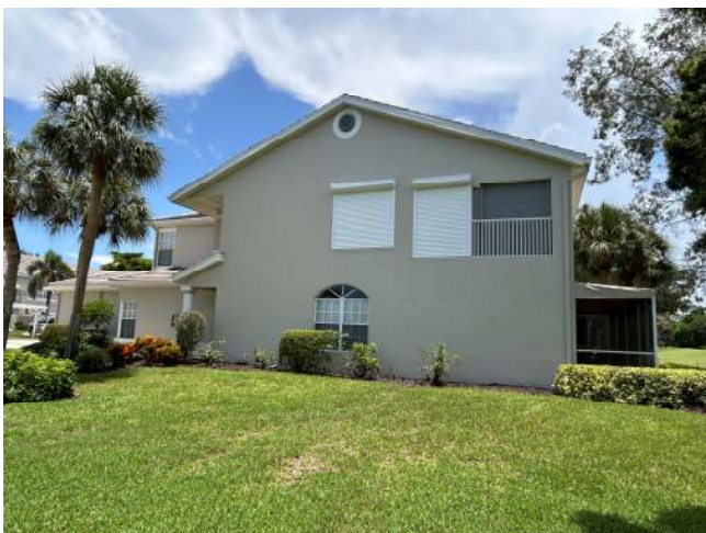
ROOF GEOMETRY – Gable / Other Roof Shape
