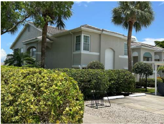
ROOF GEOMETRY – Gable / Other Roof Shape
