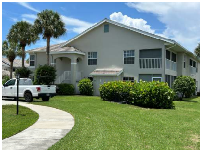
ROOF GEOMETRY – Gable / Other Roof Shape
