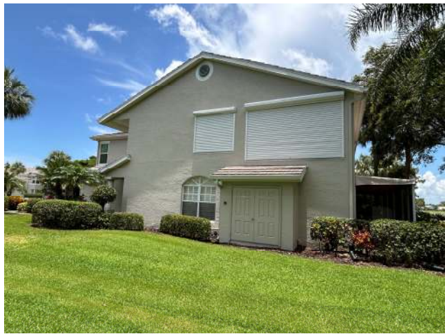
ROOF GEOMETRY – Gable / Other Roof Shape
