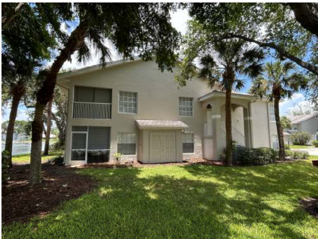
ROOF GEOMETRY – Gable / Other Roof Shape
