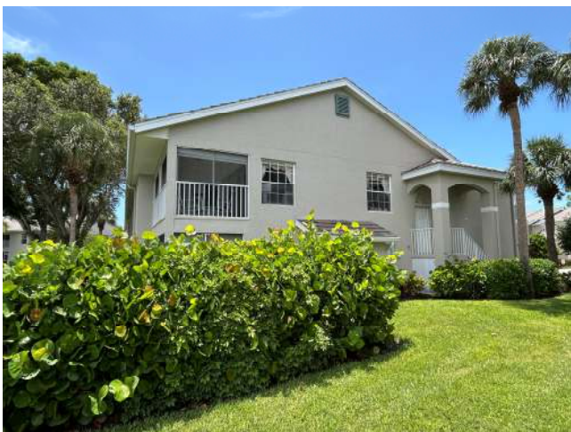
ROOF GEOMETRY – Gable / Other Roof Shape
