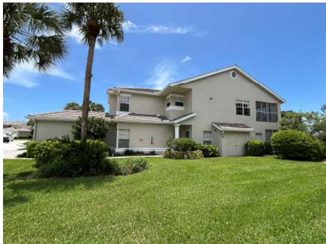
ROOF GEOMETRY – Gable / Other Roof Shape
