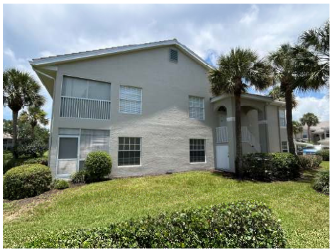
ROOF GEOMETRY – Gable / Other Roof Shape
