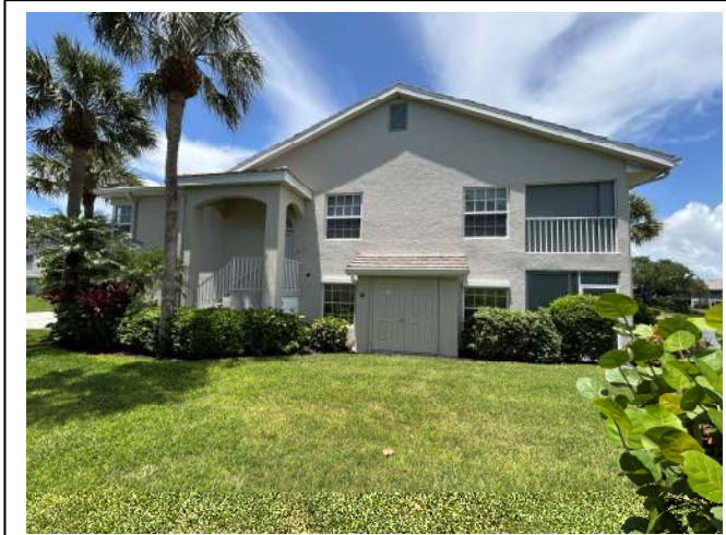
ROOF GEOMETRY – Gable / Other Roof Shape
