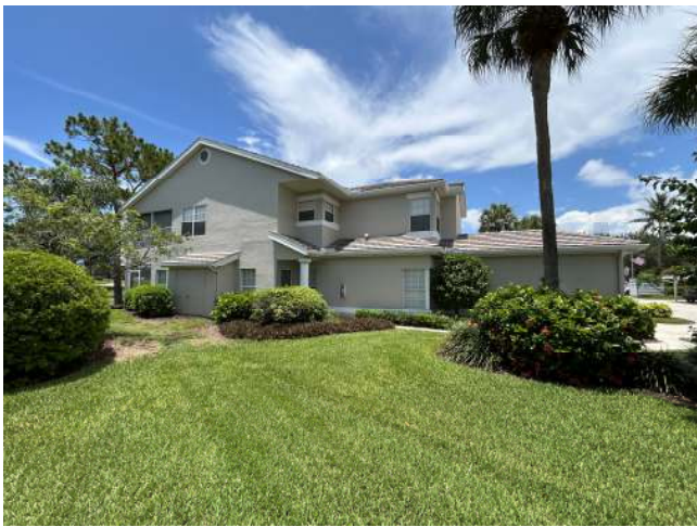
ROOF GEOMETRY – Gable / Other Roof Shape
