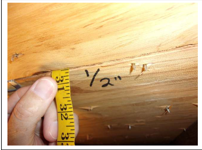
ROOF DECK THICKNESS – 15/32 to 1/2 inch plywood
