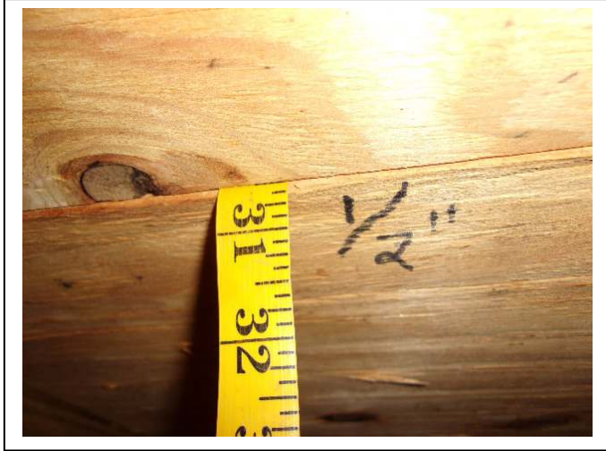
ROOF DECK THICKNESS – 15/32 to 1/2 inch plywood
