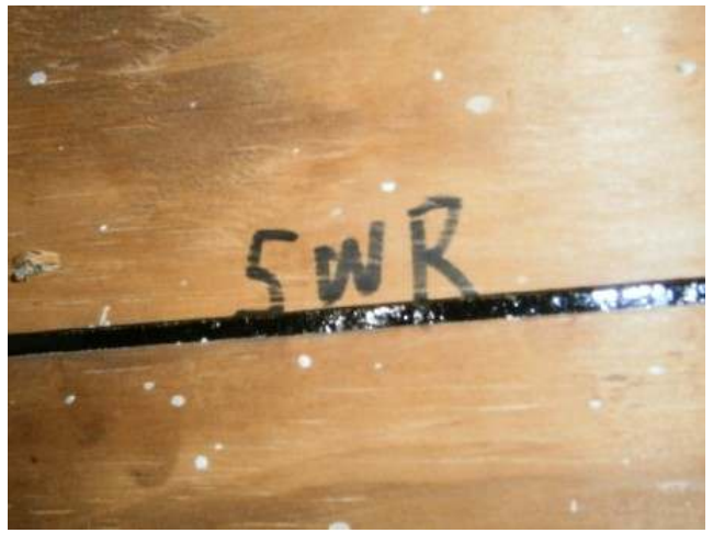
SECONDARY WATER BARRIER – A Peel & Stick adhesive polymer SWR Barrier was installed in 2014 when the covering system was replaced
