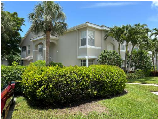
ROOF GEOMETRY – Gable / Other Roof Shape
