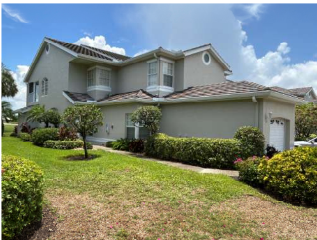
ROOF GEOMETRY – Gable / Other Roof Shape
