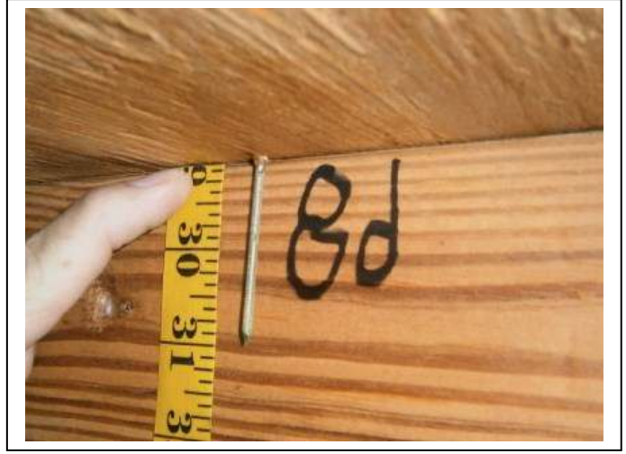
ROOF DECK ATTACHMENT – 8d ring shank nails added in 2014
