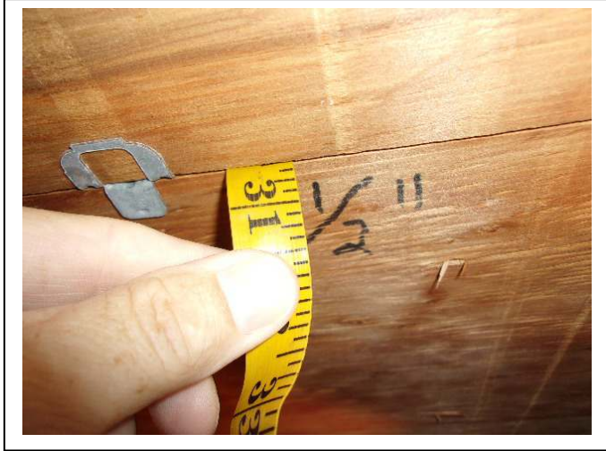
ROOF DECK THICKNESS – 15/32 to 1/2 inch plywood
