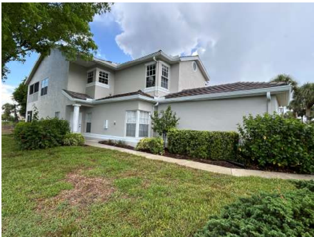
ROOF GEOMETRY – Gable / Other Roof Shape
