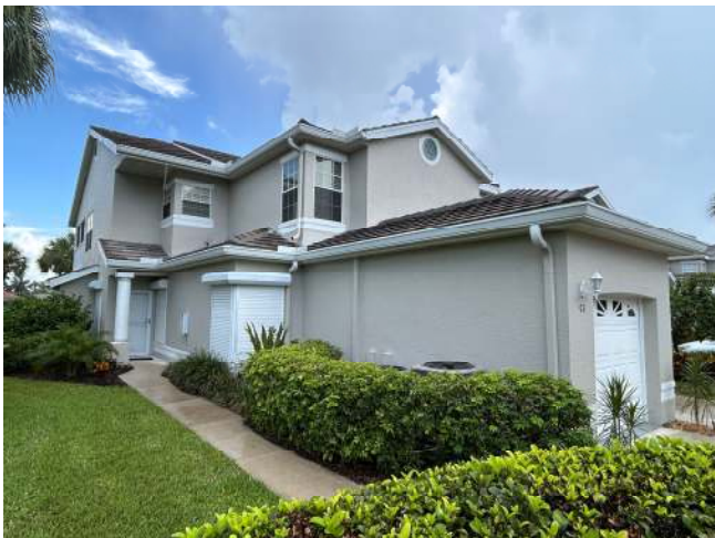
ROOF GEOMETRY – Gable / Other Roof Shape
