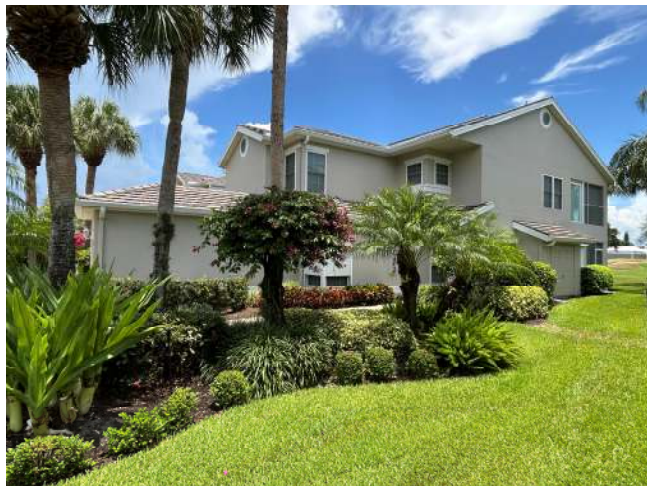
ROOF GEOMETRY – Gable / Other Roof Shape
