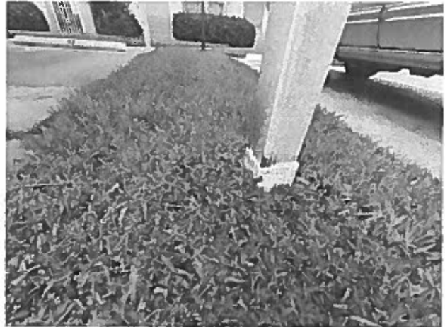
Carport structural column – deterioration of the paint finishes evident
