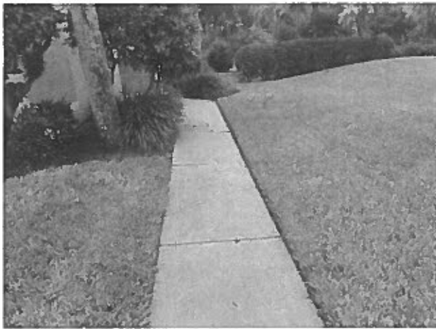
Concrete sidewalks – minor uplift evident
