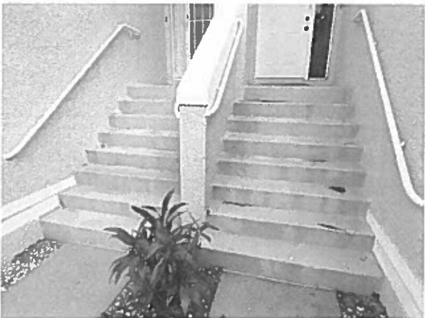
Railings – garage units – typical configuration
