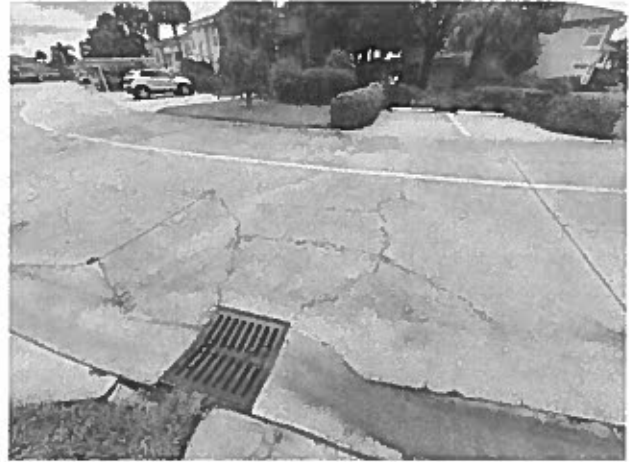
Concrete street system – cracks evident
