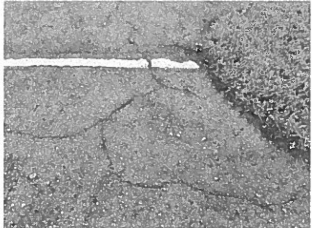
Asphalt pavement – cracks and raveling evident
