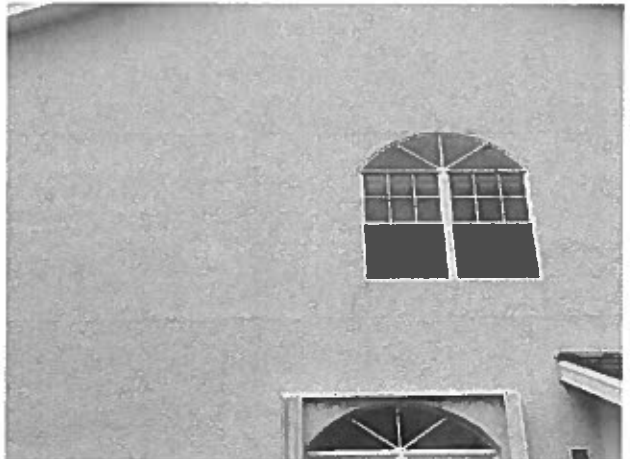
Stucco coated walls – crack repairs evident
