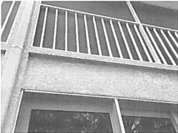
Stucco coated walls – deterioration of the stucco coatings evident
