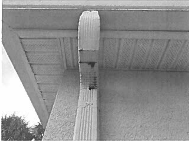
Gutters and downspouts – typical condition – deterioration of the paint finishes evident
