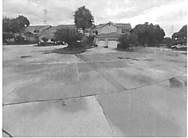
Concrete street system – cracks as well as partial concrete replacement evident – Hamilton Harbour Drive
