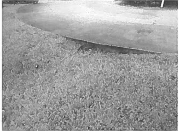
Concrete street system – erosion at Hamilton Harbour Drive evident
