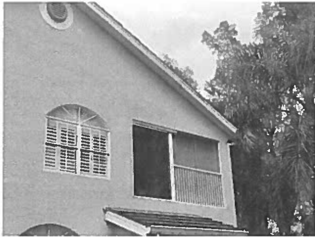
Stucco coated walls – stucco coating repairs evident as well as deterioration of the paint finishes on the fascia evident
