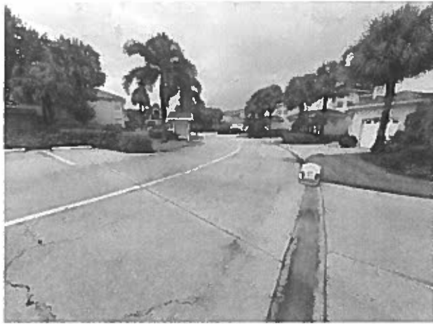
Concrete street system – cracks evident
