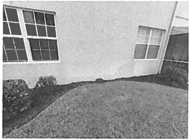
Stucco coated walls – crack repairs and deterioration of the paint finish applications evident
