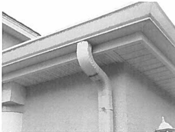
Gutters and downspouts – typical – deterioration of the paint finishes evident
