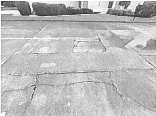
Concrete street system – cracks as well as partial concrete replacement evident
