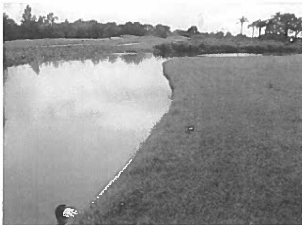
Pond shorelines – minor shoreline erosion as well as steep slopes evident
