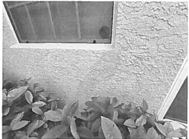
Stucco coated walls – crack repairs evident
