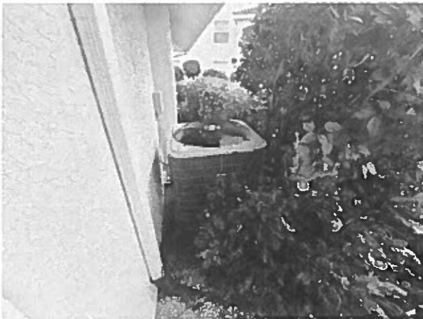
HVAC equipment – condenser unit
