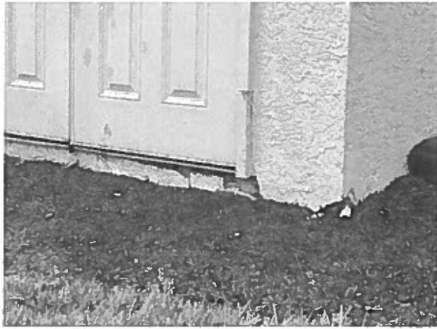
Stucco coated walls – cracks as well as stucco coatings delamination evident
