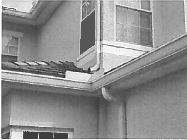
Concrete tile roofs – downspout discharging onto the roof below – this condition could lead to accelerated deterioration of the roofs
