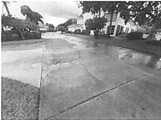
Concrete street system – cracks evident
