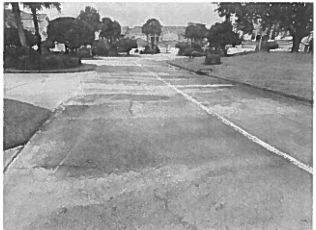
Concrete street system – cracks evident
