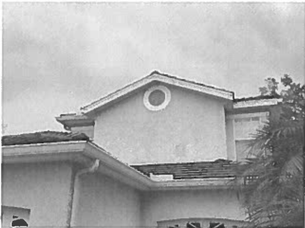
Stucco coated walls – deterioration of the stucco coatings and paint finish applications evident
