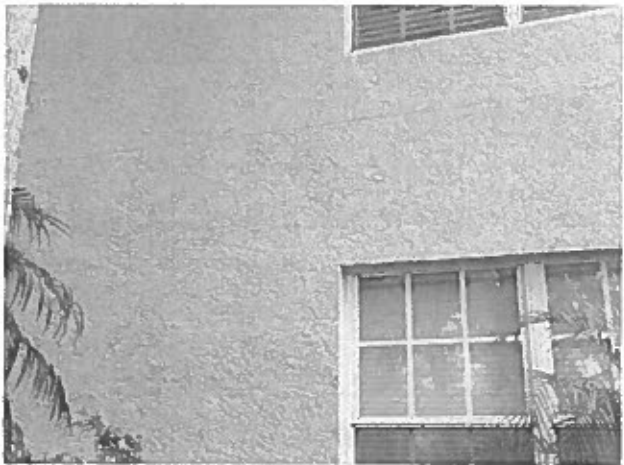
Stucco coated walls – crack repairs evident
