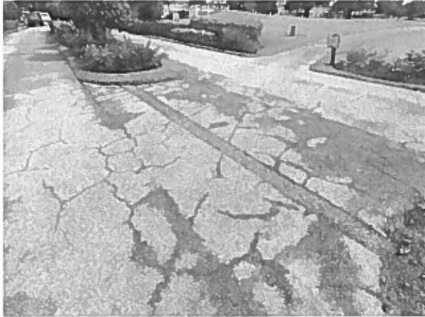
Asphalt pavement – cracks evident
