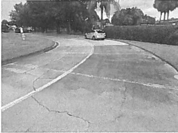
Concrete street system – cracks evident
