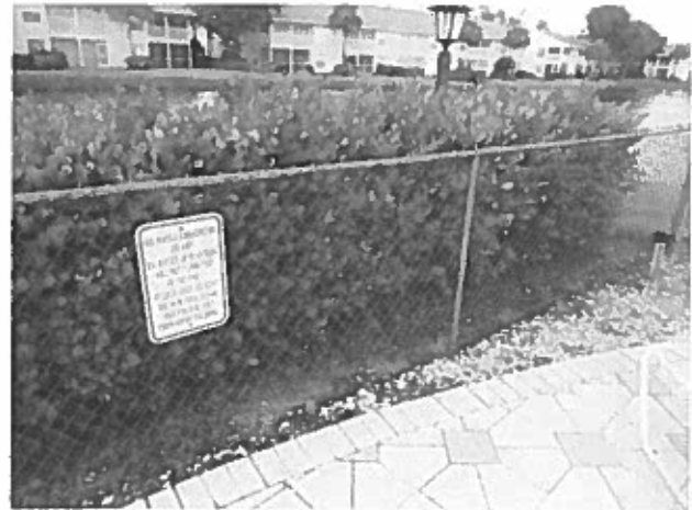
Chain link fence – overview – deterioration of the finishes evident
