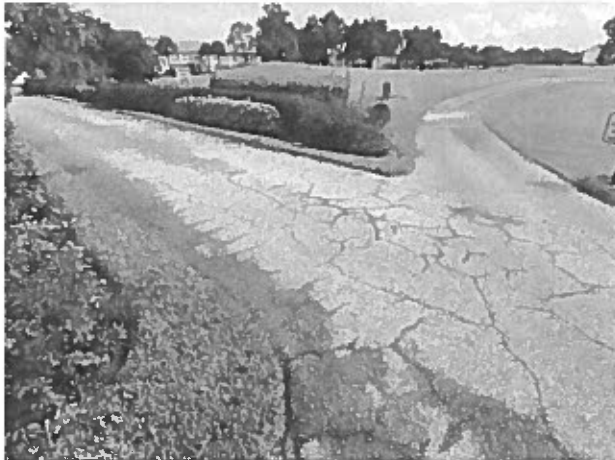
Asphalt pavement – cracks evident
