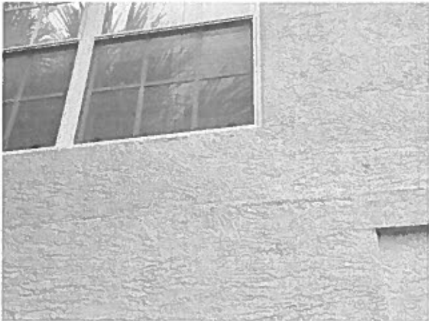
Stucco coated walls – crack repairs evident
