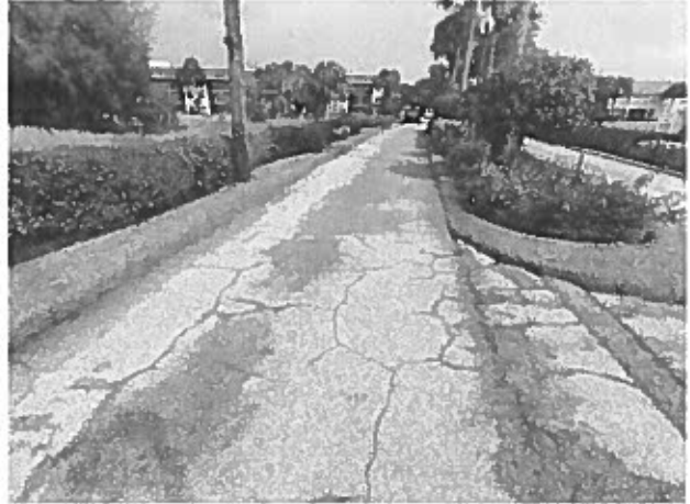
Asphalt pavement – cracks evident
