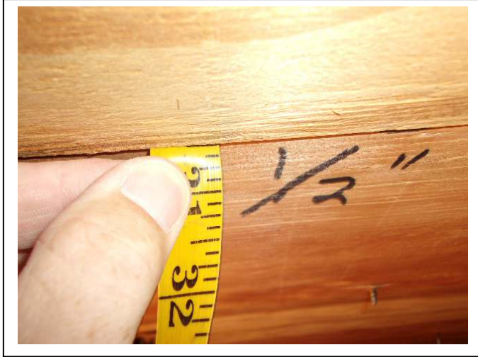
ROOF DECK THICKNESS – 15/32 to 1/2 inch plywood
